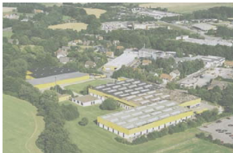
Kannegiesser Works at Vlotho
